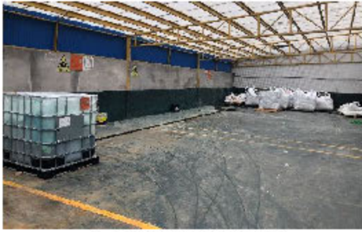
(a) 危废仓库内导流沟
