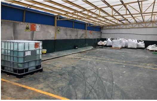
(a) 危废仓库内导流沟
